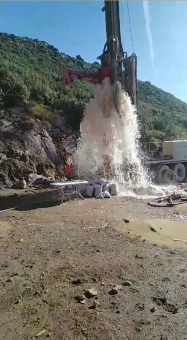
Annexe 2 : Drilling Development Test Phase (march 2020)
