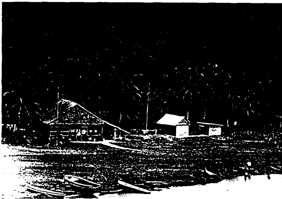
Figure 9. Field headquarters in Rio Belen: main field house (left), compressor and generator shed (center), and fuel depot (right). The single side band radio aerial is stretched between two tall poles in front of the house.
