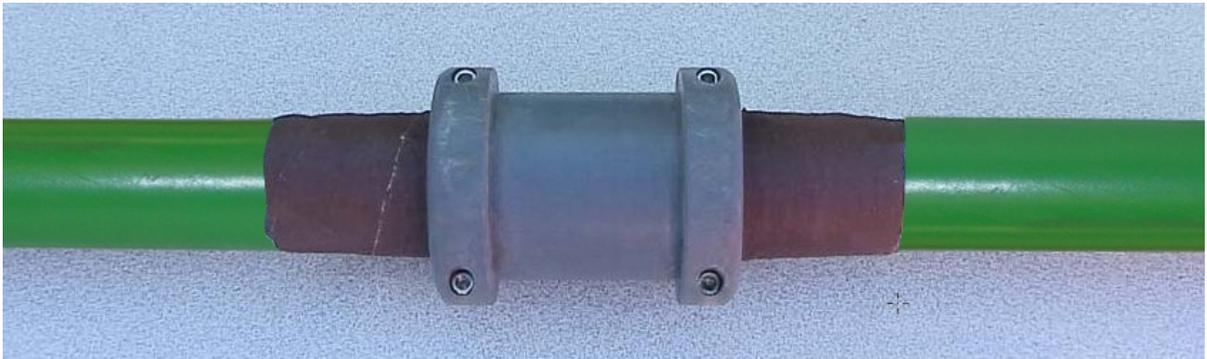
Figure A118: Bird collar installed.
