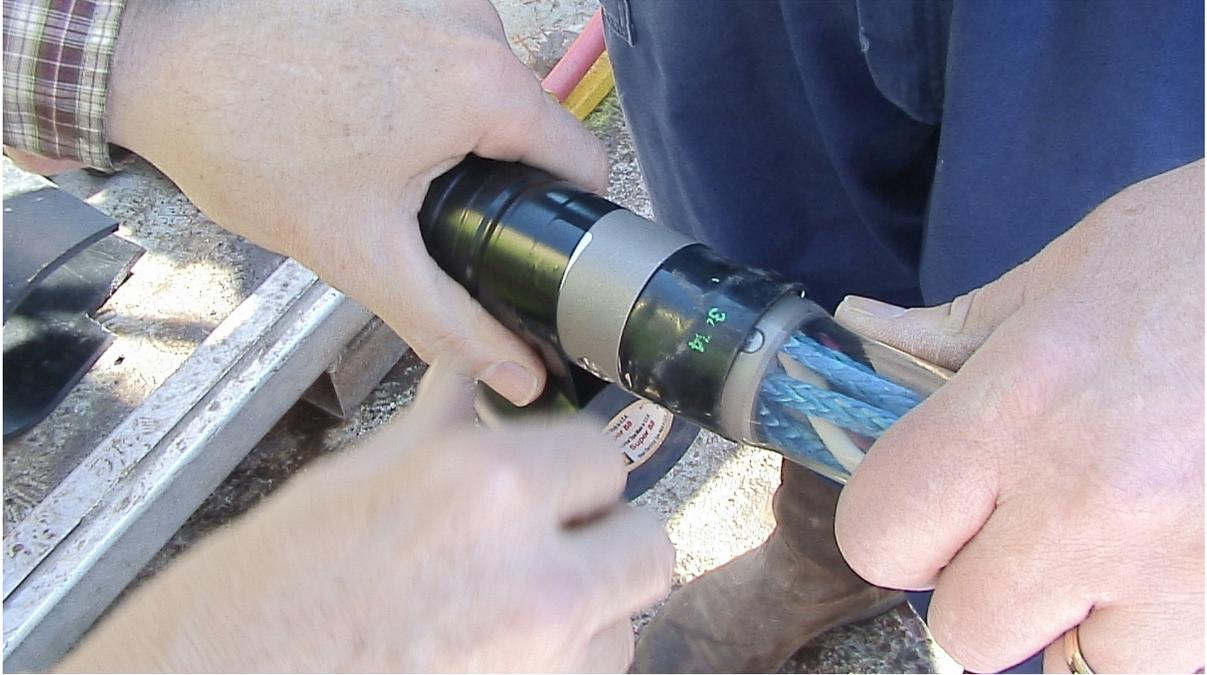
*Figure A110: Applying tape to connector to prevent loosening.*
