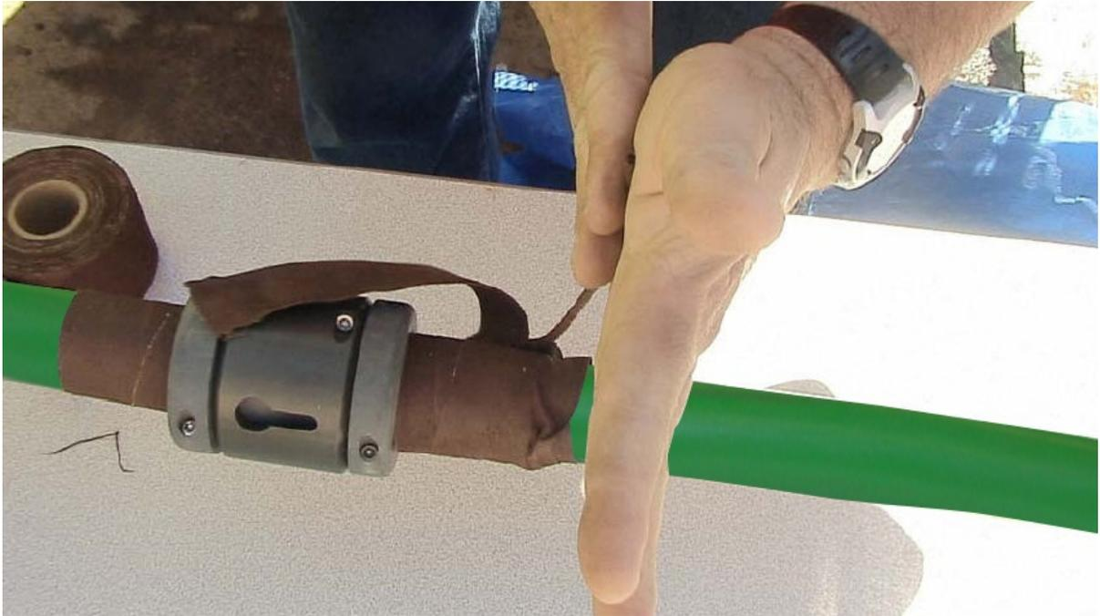
*Figure A128: Preparing friction tape for tie-off.*
