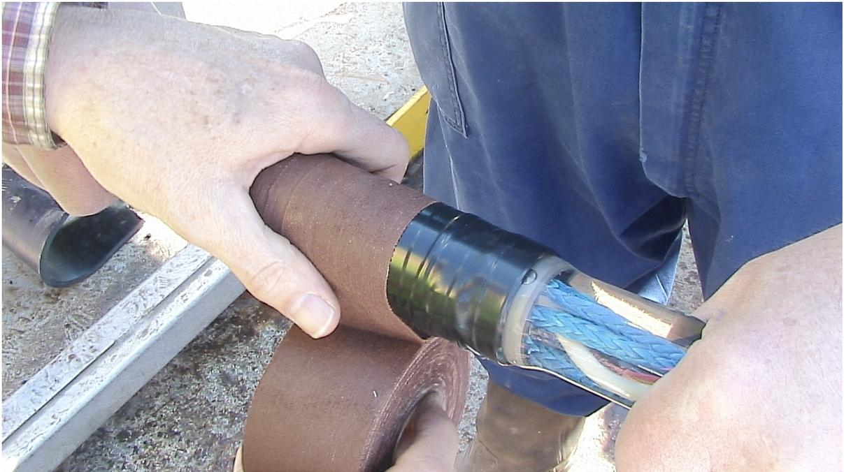
*Figure A111: Applying friction tape over electrical tape on connector.*
