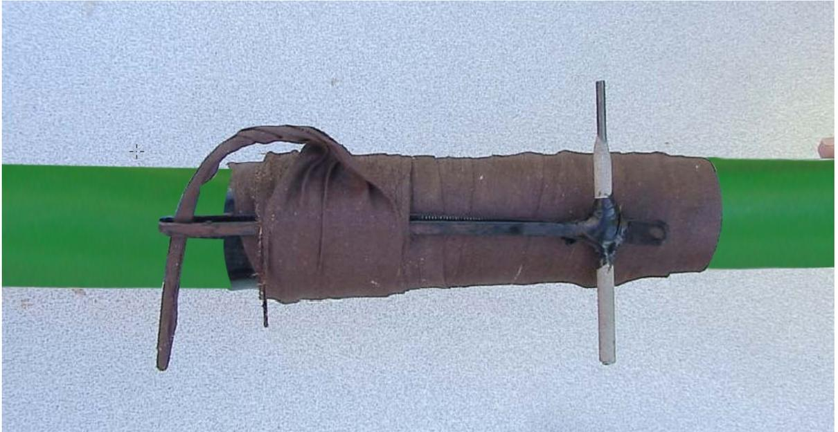
*Figure A133: Friction tape "tail" ready to be pulled.*
