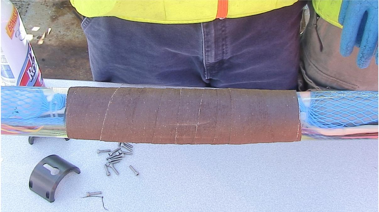
*Figure A117: Installing friction tape as part of collar installation.*
