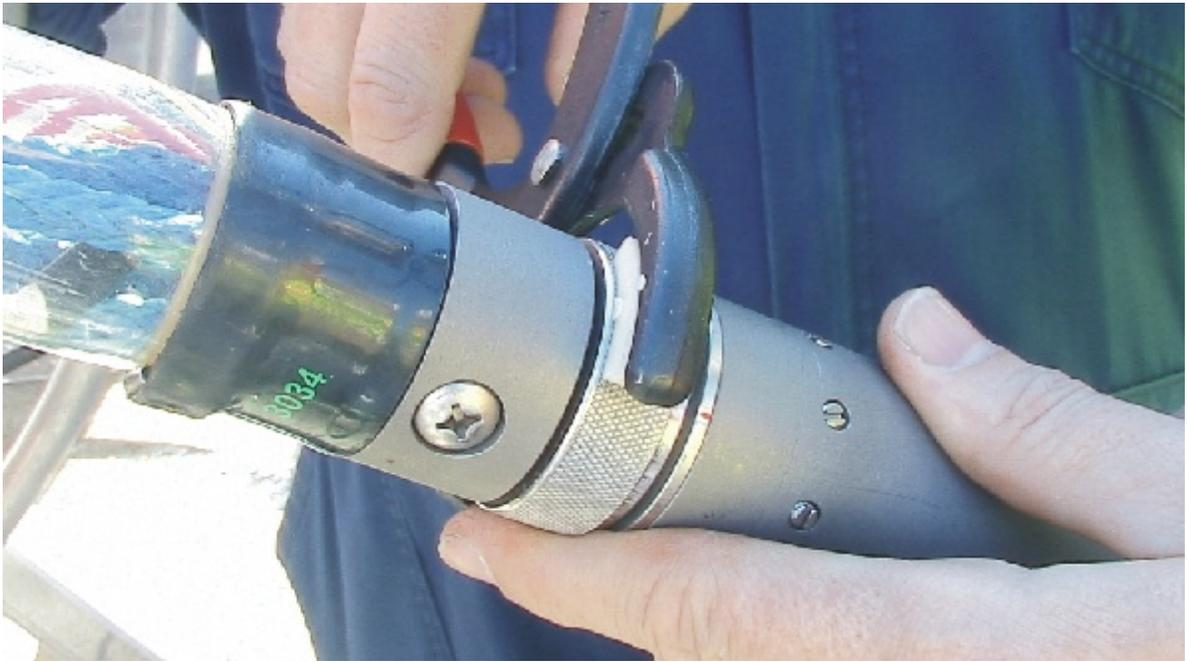
*Figure A109: Securing a connection with soft-jawed pliers.*
