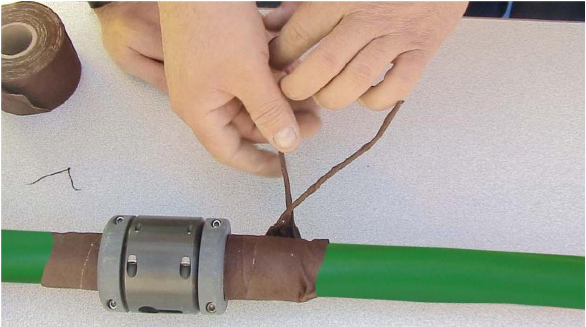
*Figure A129: Tying off friction tape.*
